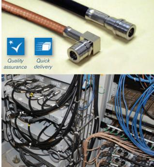
DAS installation using QMA cable assemblies.
