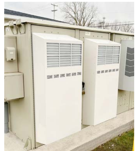
The NEMA 4-rated DualXchange DAC features a streamlined profile.
